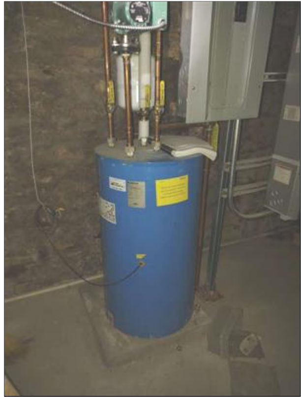
D. Picture 2 Storage Tank
