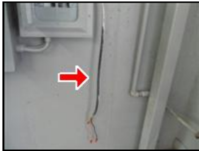
3.2 Picture 4 Wires On Wall / Capped
