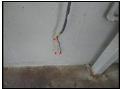
3.2 Picture 6 Improperly Terminated
