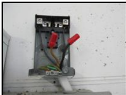
3.2 Picture 4 Wires On Wall / Capped
