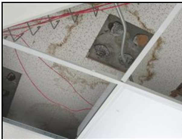
C. Picture 1 2 Layers of Ceiling Tiles
