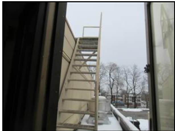
E. Picture 2 Stairs to Roof
