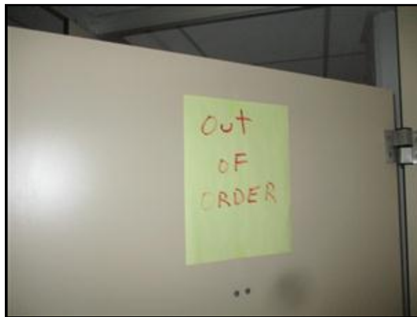
E. Picture 7 Out of Order Toilet Stall
