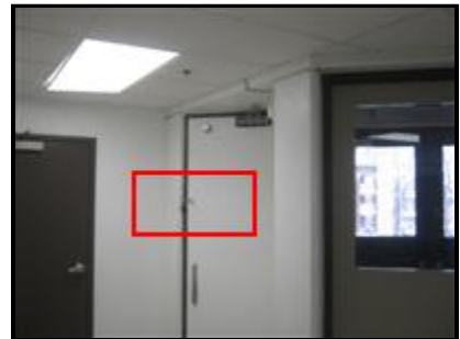
B. Picture 11 Padlock on Hall Stairwell
