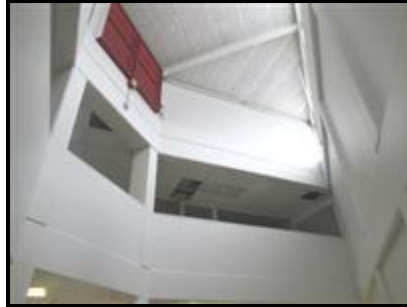
C. Picture 2 1st floor view to 2nd Floor
