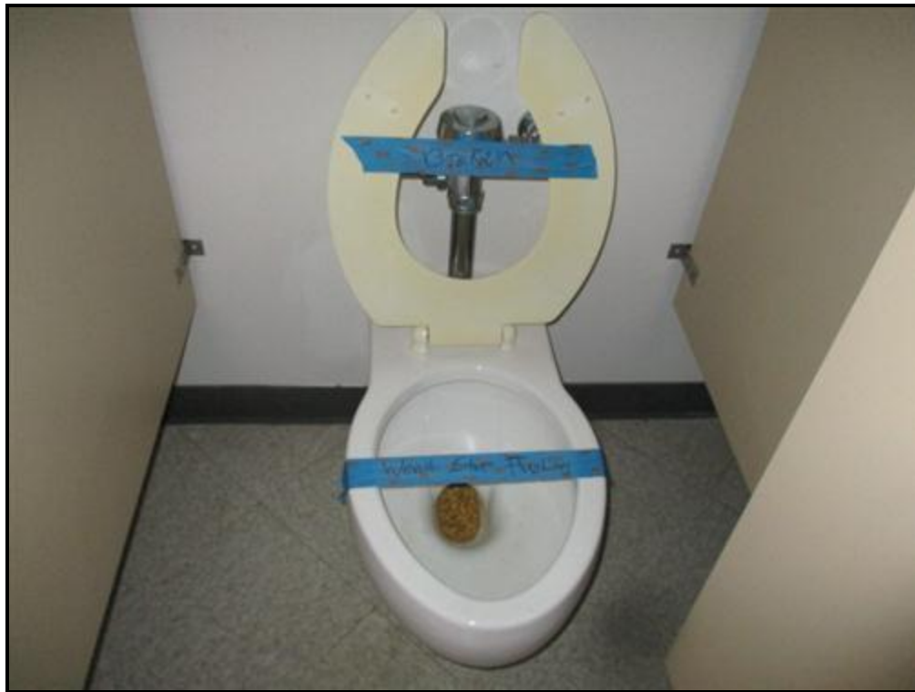
E. Picture 8 Won't Stop Flushing / Broken Seat
