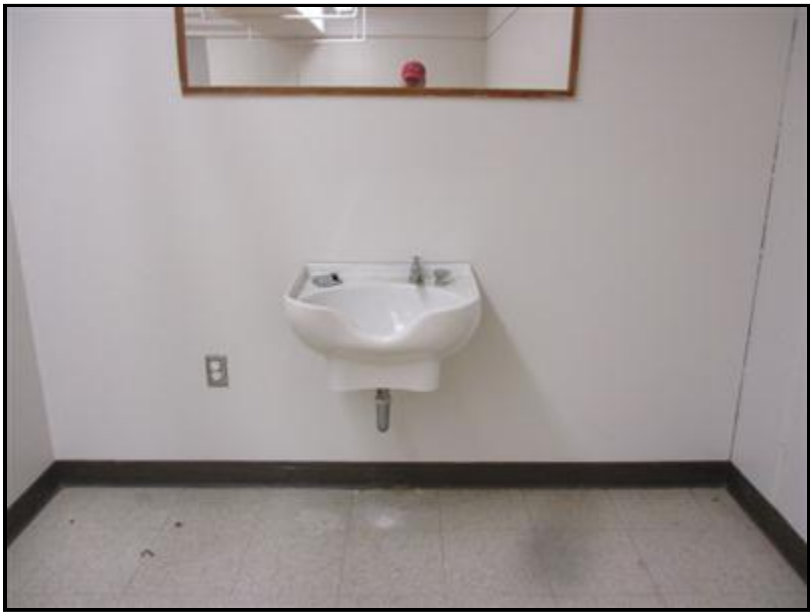
E. Picture 15 Leaks
