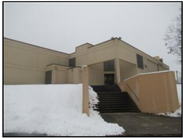
A. Picture 6 Front Entry Stairs
