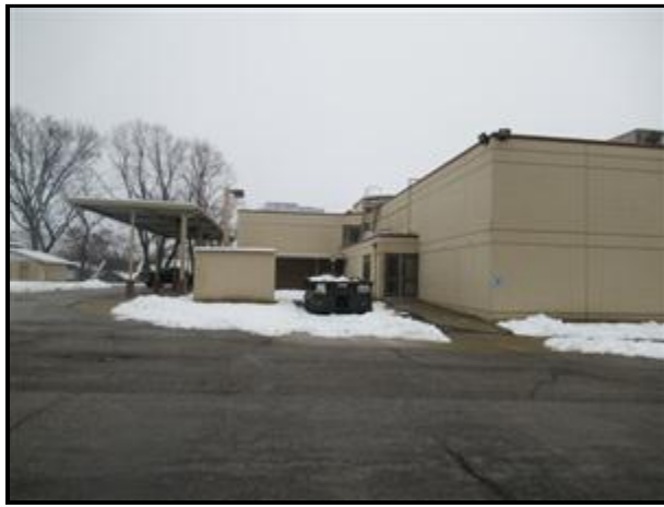
A. Picture 5 Covered Parking Canopy
