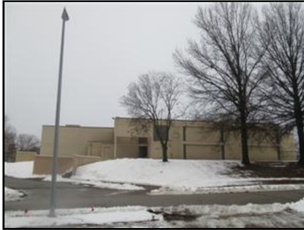
A. Picture 1 Front of Bldg / West
