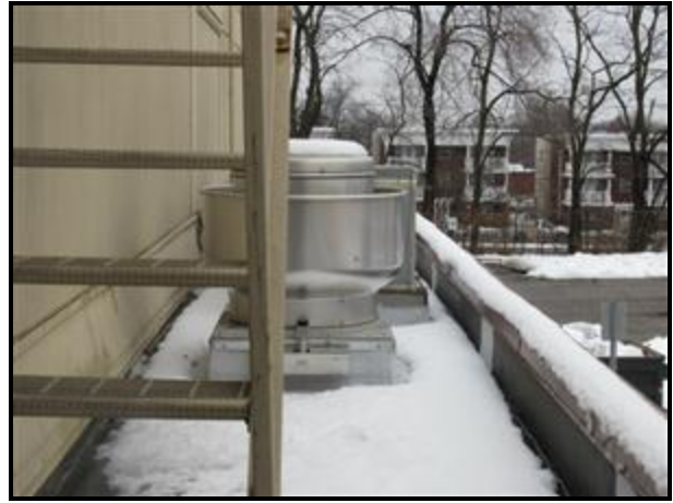
E. Picture 4 Lower Roof & Parapet Flashing
