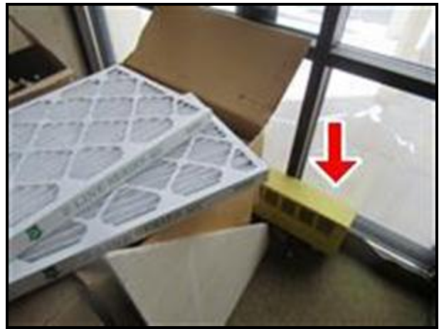
F. Picture 9 Filter Room
