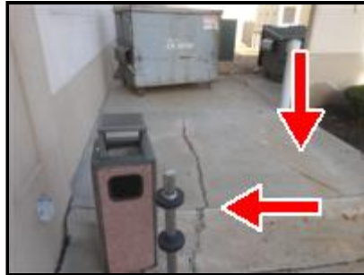
F. Picture 8 Rear Bldg by Trash Containers
