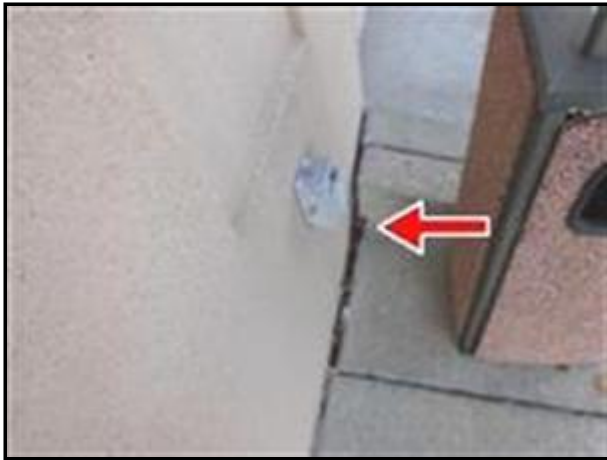
F. Picture 1 Rear of Bldg by Service Door
