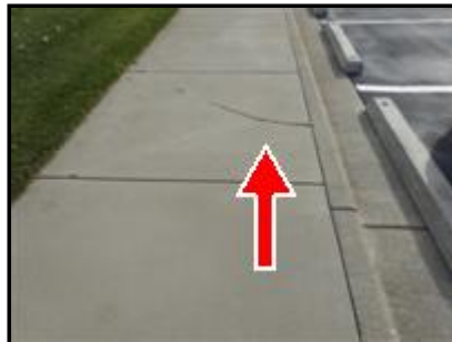
F. Picture 6 Front of Bldg
