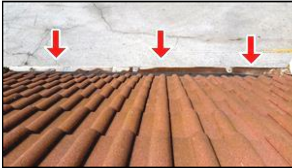
7.3 Picture 1 From Flat Roof Looking Down
