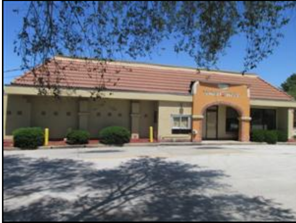
8.3 Picture 4 Drive Thru Window / West Entry
