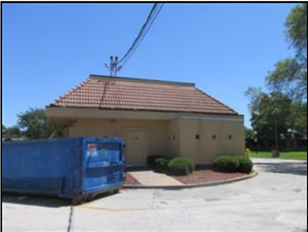
8.3 Picture 3 Rear of Building
