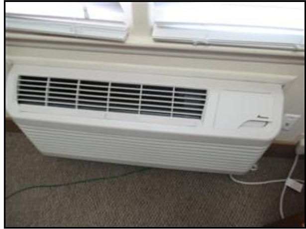
5.0 Picture 2 PTAC Thru Wall Unit
