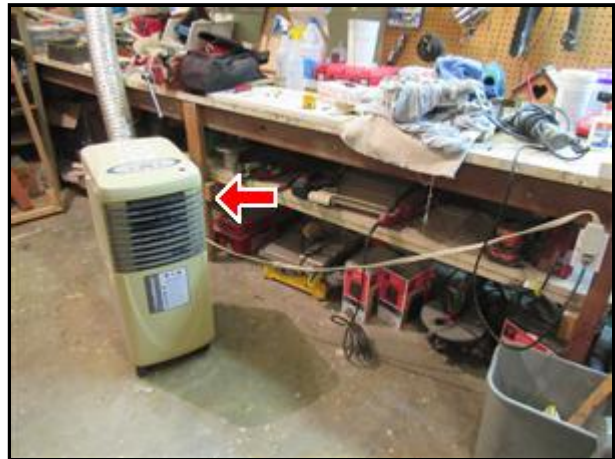
5.0 Picture 4 Basement Work Shop
