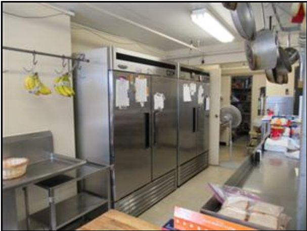
1.0 Picture 4 Refrigerator / Freezer
