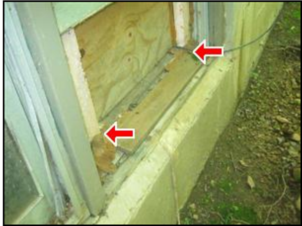
9.1 Picture 2 Window Sills
