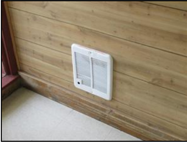
5.0 Picture 1 Electric Heater / No Knobs
