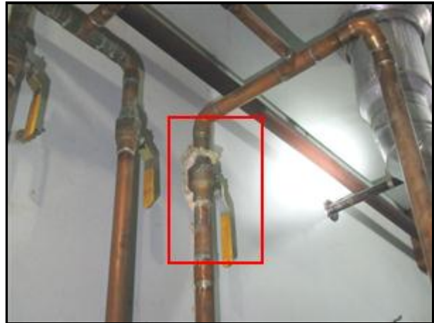
3.5 Picture 2 Corrosion
